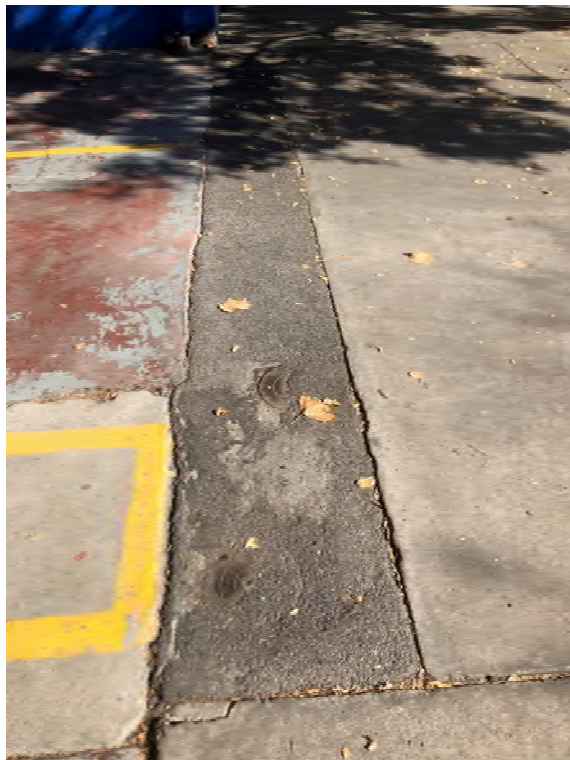
Photo 4: Potential UST fill point
